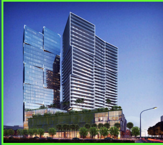
One West Palm Construction started 200 rooms
