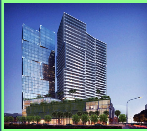
One West Palm Jeff Greene Under construction 206,706 sf
