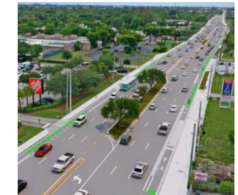
LAKE WORTH RD. RESURFACING PROJECT
