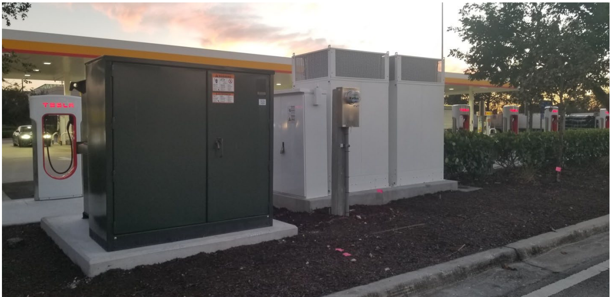
Figure 21 Electrical equipment for BEV charging station at Florida Turnpike Lake Worth service plaza from north side looking south. This area could easily be used to double the charging stations when needed. Gulf service station in the background with gasoline pumps approximately 60 feet away.
