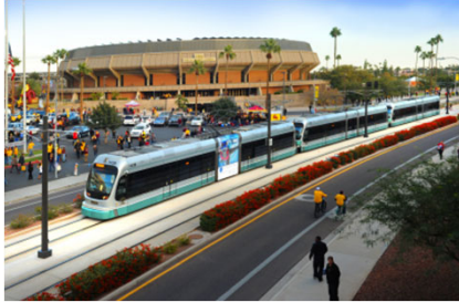
Primarily operates in dedicated rail lanes
